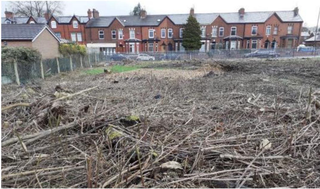
Photo 5: Looking out of the site
